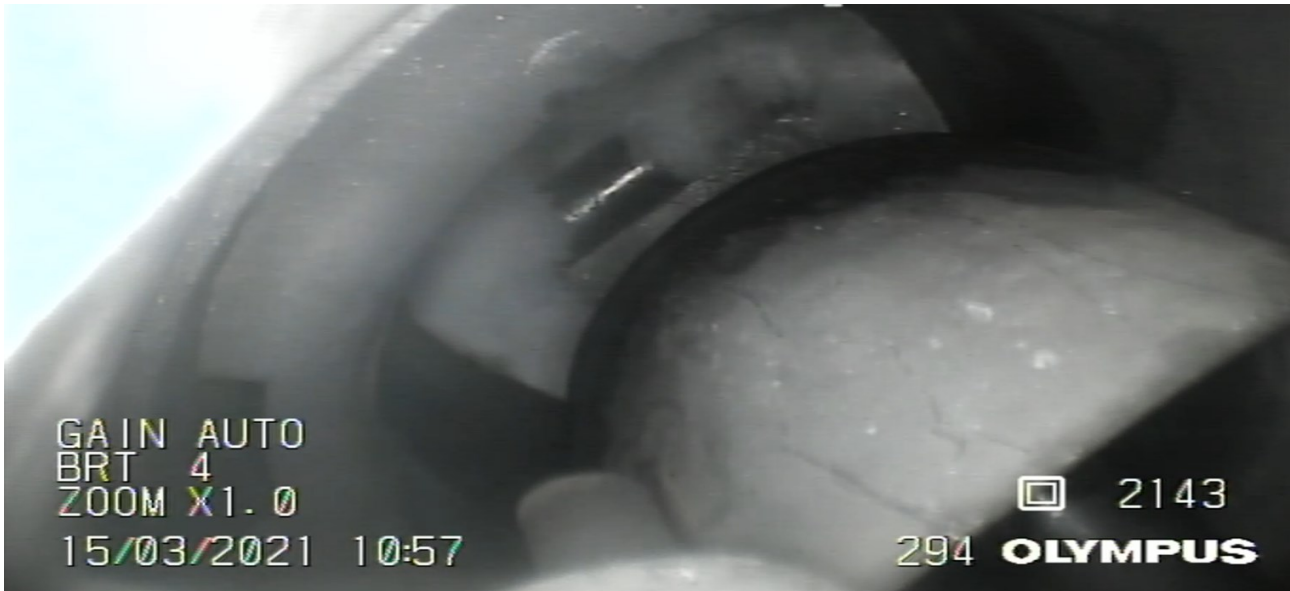
Figure 114: progress of icing => initiation of phase five => time designated t_4 Source: BEA
