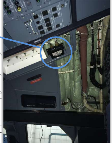
Pre-amplifier (CU hidden under a cover panel).
