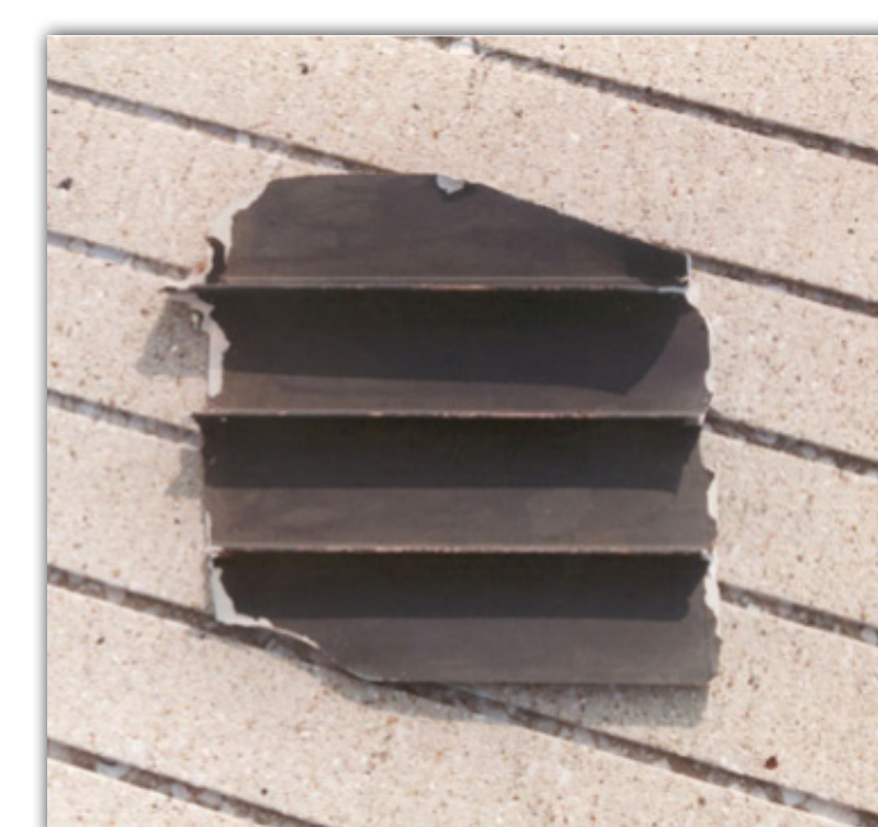
Part of tank No. 5
