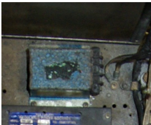
Figure 36: Circuit breaker in position on the cockpit floor and not electrically connected
