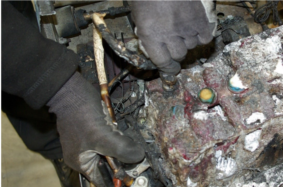
Figure 55: Repositioning of conductor on positive terminal of battery Source: BEA
