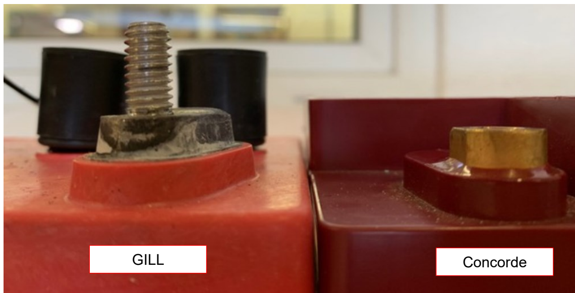
Figure 46: Comparison between a GILL battery terminal and a Concorde battery terminal Source: Flugschule Basel AG
