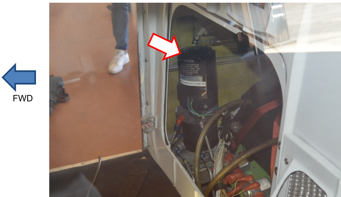
Figure 24: Hydraulic pump Source: BEA
