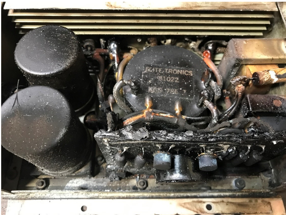
Figure 34: Components of 12 V - 24 V converter Source: BEA
