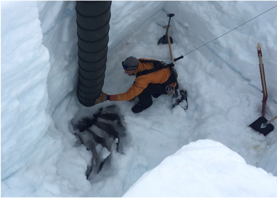
Fig. 44: Photo by Dirk van As, Greenland Guidance. Photo of Icelandic rescuer melting out fan hub
