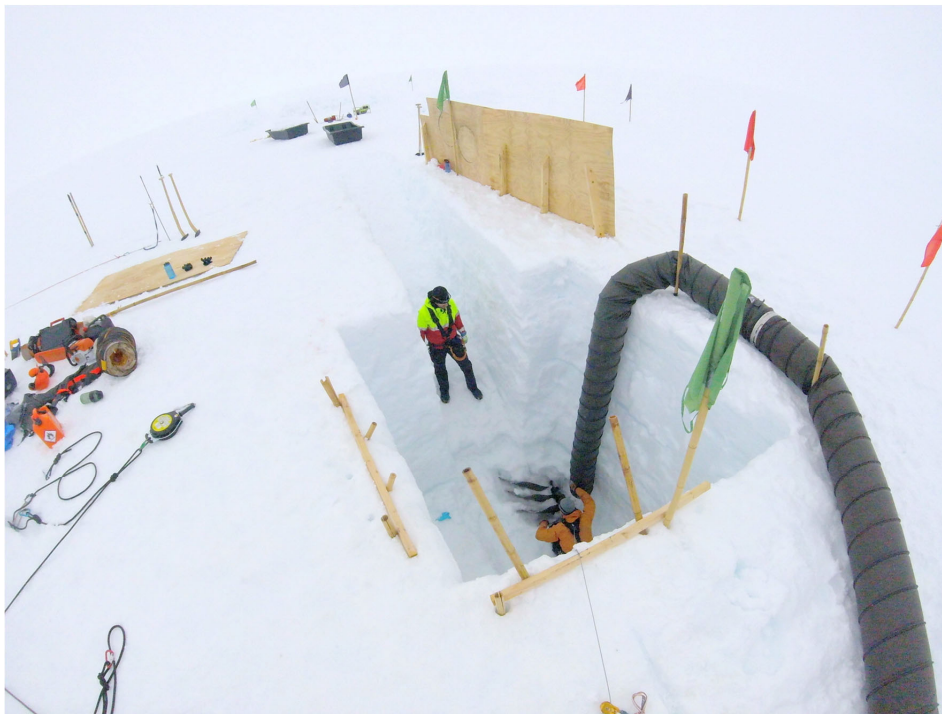
Fig. 43: Melting out snow and ice around part in 4 m deep hole. Photo by Arnar Ingi Gunnarsson
