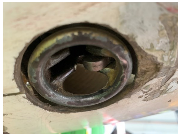
Figure 4: hook in OPEN position (source: BEA)
