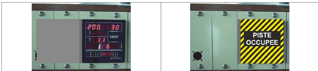
Figure 2: wind indicator and masking panel (source: Melun-Seine OM)
