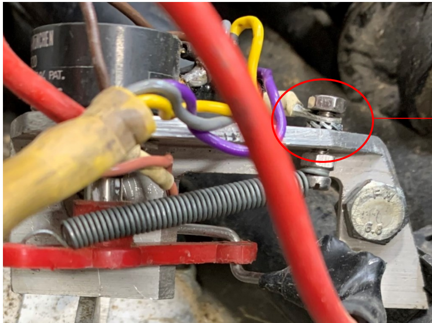
Figure 3: ground conductor lug not tight (source: BEA)
