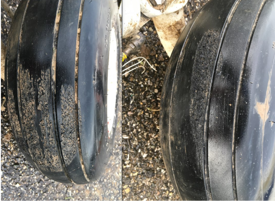
Figure 1: reverted rubber mark on left and right main gear tyres (Source: BEA)
